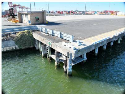
As part of our stewardship obligations, Port of Melbourne has commenced remediation works of timber piles at Appleton Dock. These pile works will ensure the safe operation of the wharf without any load restrictions into the future. Since December 2024, our contractor Bhagwan Marine has completed 23 pile repairs out of a total 224.
