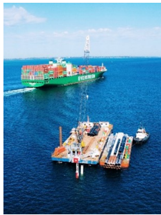
A total of 29 beacon piles will be replaced throughout Stage One of the project without
