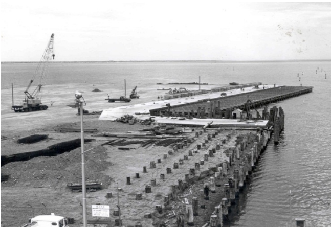
Webb Dock under construction
